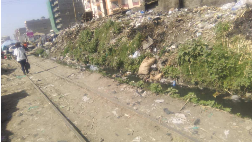
Part of the existing Pipeline Railway
