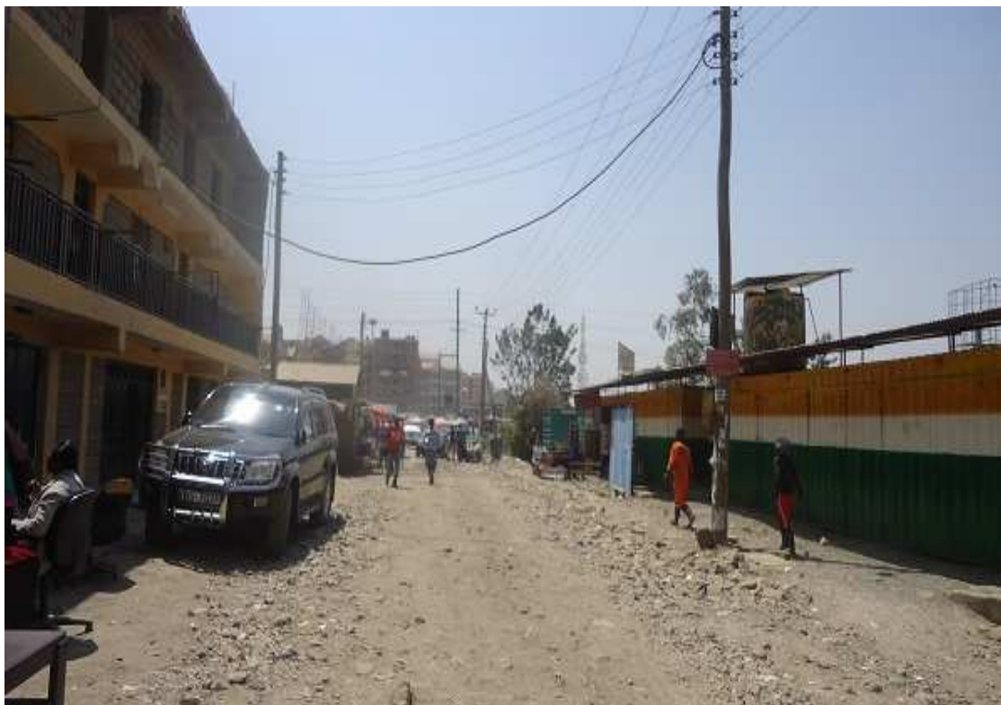
Figure 4-3: Electricity supply within Pipeline Estate
