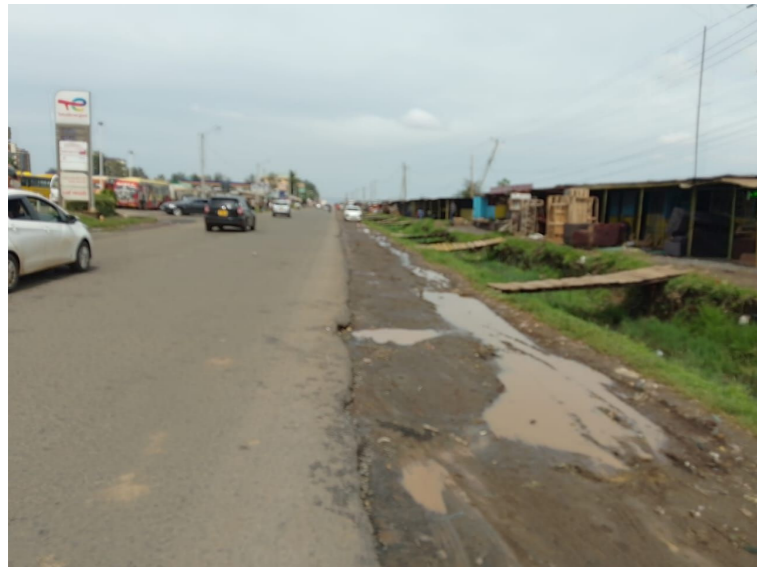
VIEW OF STORM WATER DRAIN ALONG MWIKI - KASARANI ROAD
