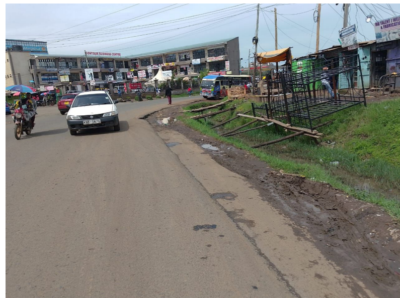
SITE FRONTAGE ALONG KASARANI - MWIKI ROAD
