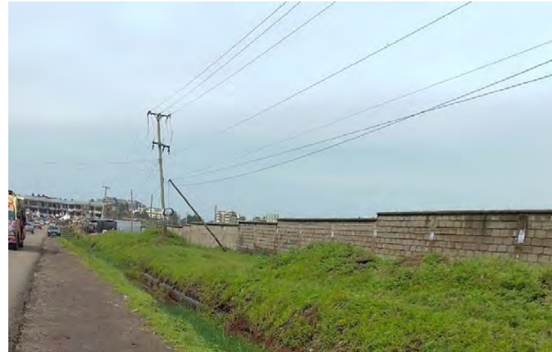
VIEW OF POWER LINE ALONG THE SITE BOUNDARY
