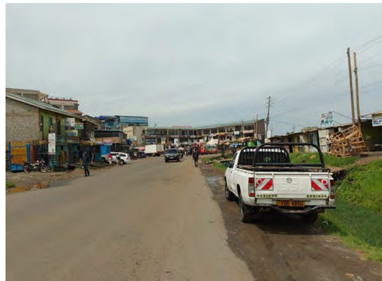
VIEW OF KASARANI - MWIKI ROAD
