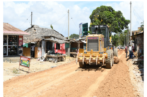
Ongoing Slum Upgrading Works in Kilifi County
