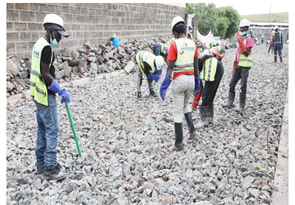
KISIP2 undertaking Slum Upgrading Works in Nakuru's London - Hilton informal settlement
