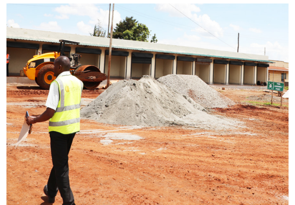
Ongoing development of modern vendor platforms in Mosoriot, Nandi County
